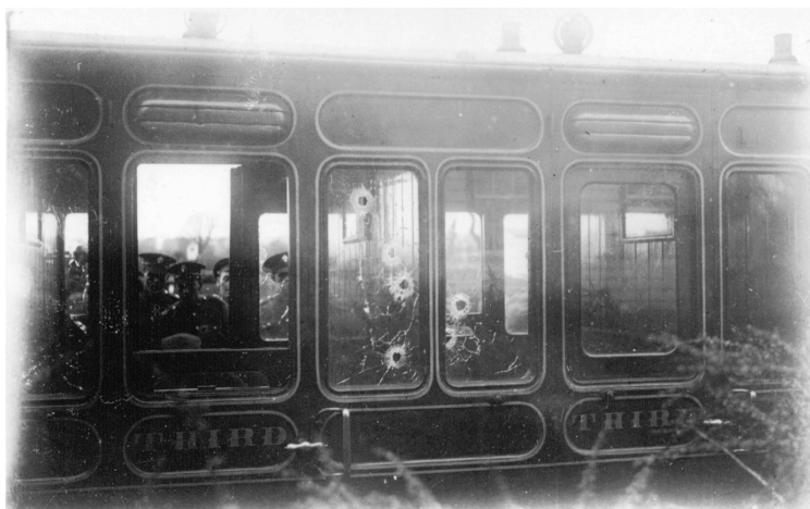
Above: The train afterwards, 3rd class 6-wheel carriage No. 663 at Tralee Bay platform, blood-stained and with bullet holes, Saturday 12 February 1921. The platform side of the coach with substantial window damage. (Photo: Museum of the Royal Fusiliers, HM Tower of London)
